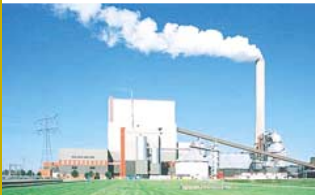
The Amer biomass co-firing power plant in the Netherlands. (Courtesy Essent, the Netherlands)
