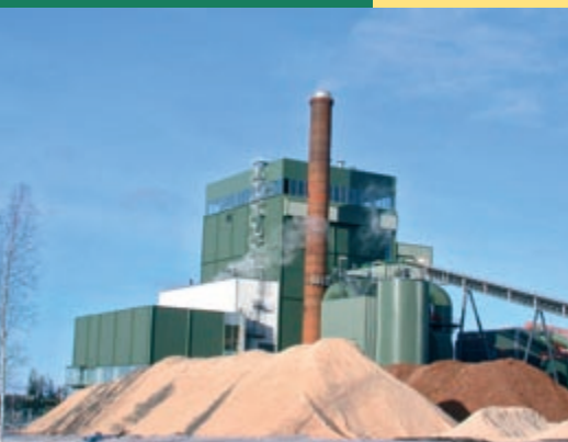
Biomass fired CHP plant in Osterson, Sweden.
